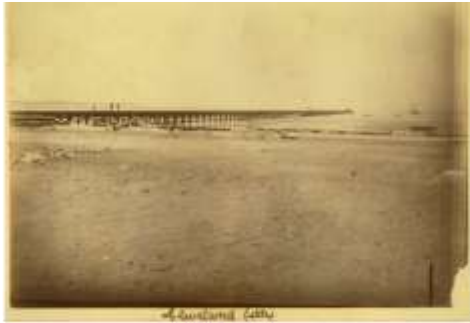
Cleveland Point jetty at Cleveland, circa 1880 (State Library of Queensland)
